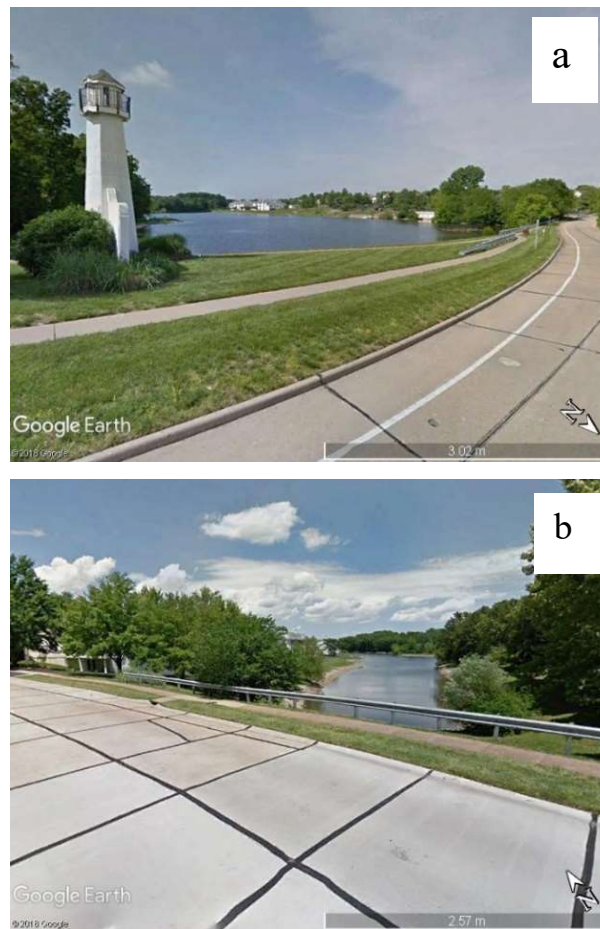
Figure 1.2. Lake Chesterfield Dams: (a) View of the North Dam. (b) View of the South Dam.
